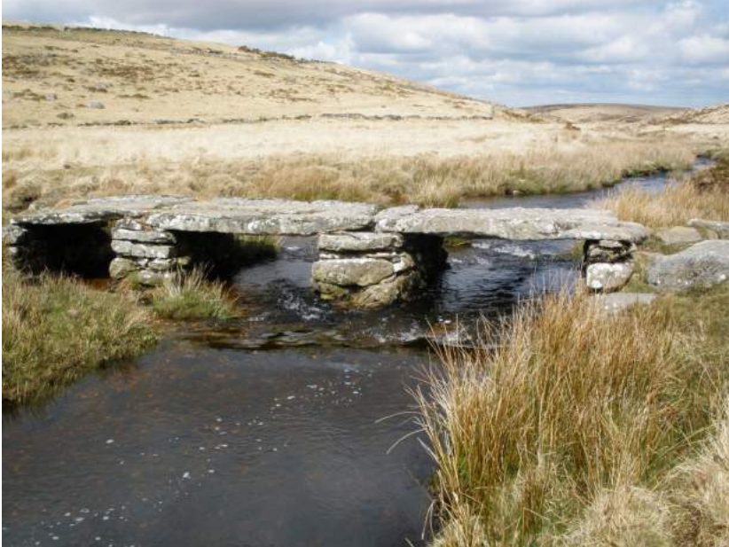
Plate 94. The clapper bridge across the North Teign, near the derelict farms at Teignhead and Manga.
