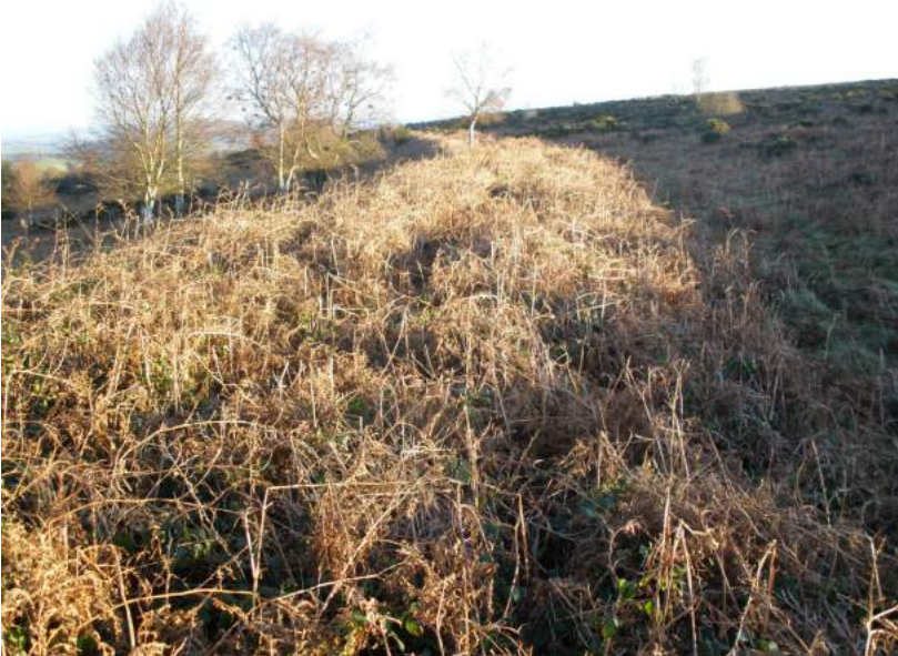
Plate 49. The embankment of the railway line built in 1943-4 by U.S. Army.
