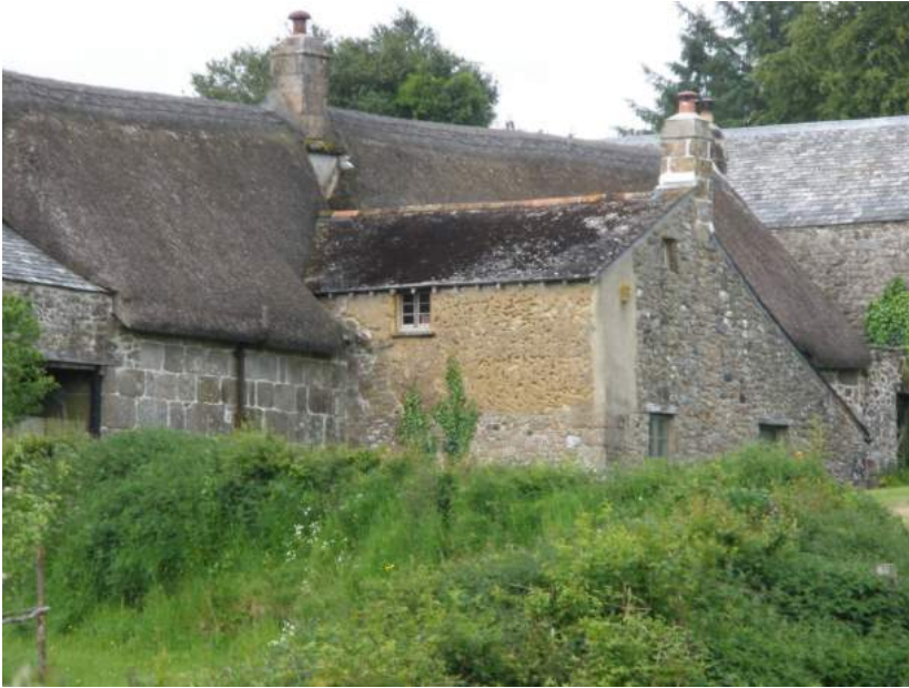
Plate 86. An incongruous juxtaposition of ashlars [the large, rectangular stone blocks] and brownish cob [puddled earth].
